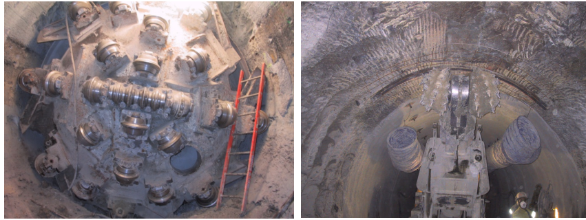
Fig. 6.5: TBM (Gripper) type machine (left). Roadheader type machine (right)
