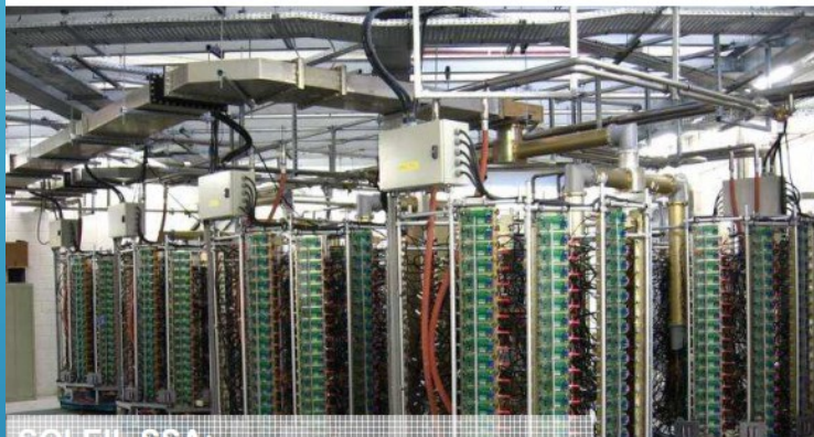
SOLEIL SSA: Frequency: 352 MHz Output power: 180 kW 726 × 315 modules in 4 towers. 2 × Si LDMOS transistors per module
